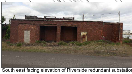
2. Redundant Riverside 2.75kv substation
