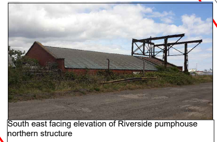
5. Riverside pumphouse northern structure, plan area = 295m 2
